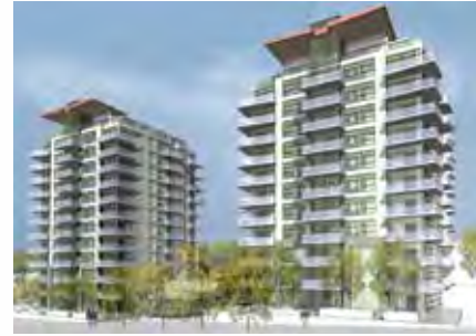
ATRIUM EAST & WEST
